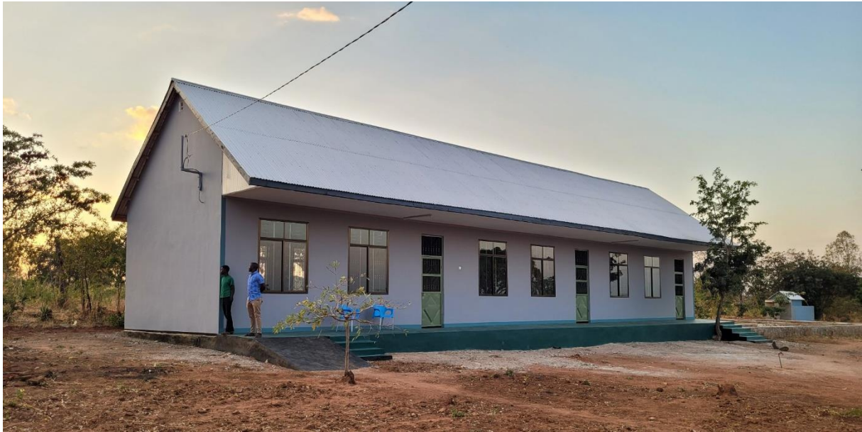
Figure 9: The Front of the Classroom Building
