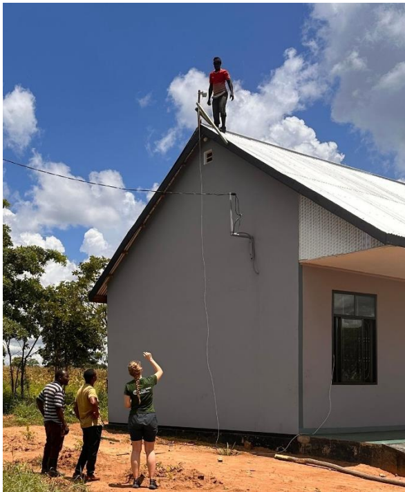
Figure 14: During the installation of the antenna. Note: Provided by the author (2024).
