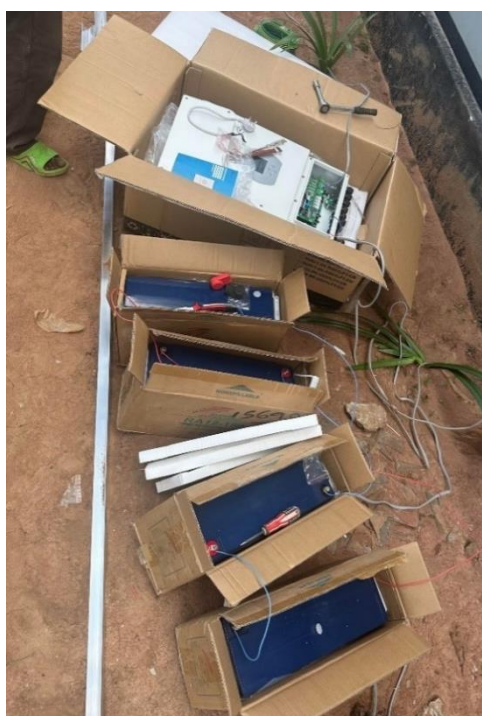
Figure 12: Hand tools were powered by batteries during a power outage. Note: Provided by the author (2024).
