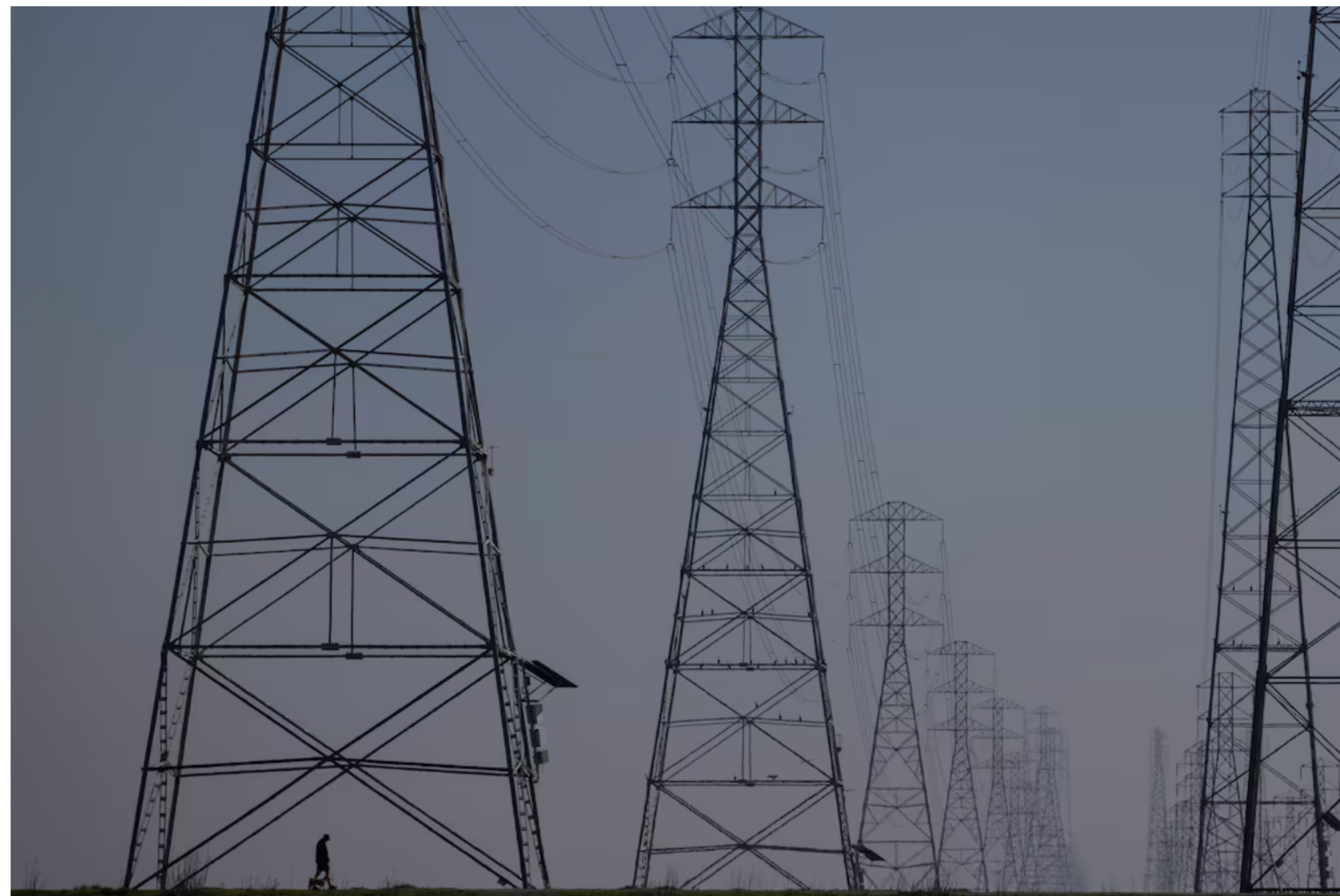
A local resident walks by the power grid towers at Bair Island State Marine Park in Redwood City, California, United States, January 26, 2022. REUTERS/Carlos Barria/File Photo Purchase Licensing Rights
