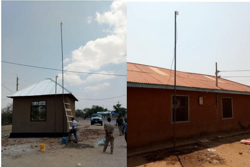
Figure 8. Izazi village office to the left and Izazi dispensary to the right. The equipment on the pole at the village office receives and sends out signals to the additional InfoSpot in the dispensary, five kilometres away. (Photos: Felix Sukums)
